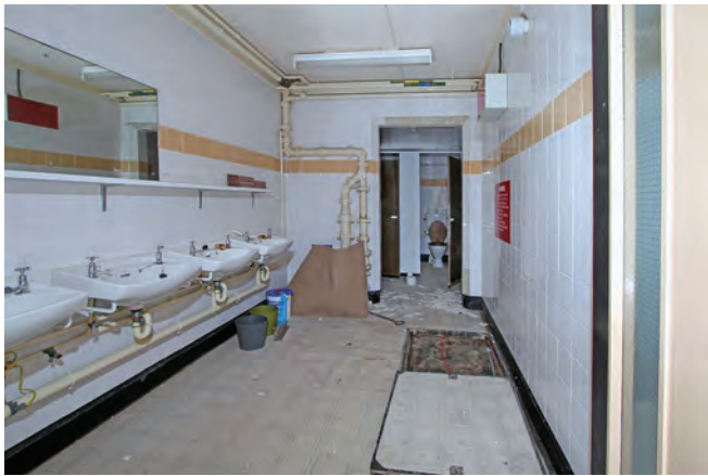
The lower floor ladies washroom and WC cubicles
